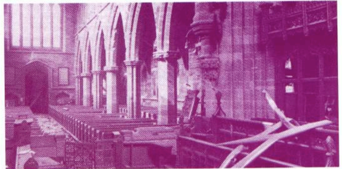
Interior of Mossley Hill Church after bomb damage
